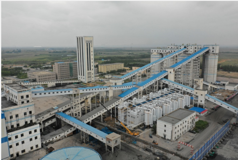
-30mm Mixed Coal Separation (9.0 Mtpa Shanghaimiao No 1 Coal Mine )
